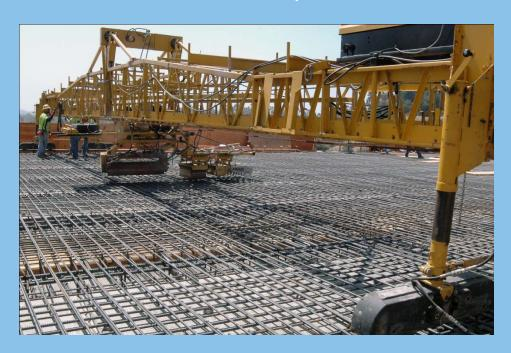
In this view looking southwest, workers finish the rebar support for the bridge deck. The new Sunset Bridge deck will be several feet higher than the current bridge deck.
